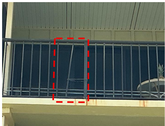
Figure 7. Missing picket at unit F12
