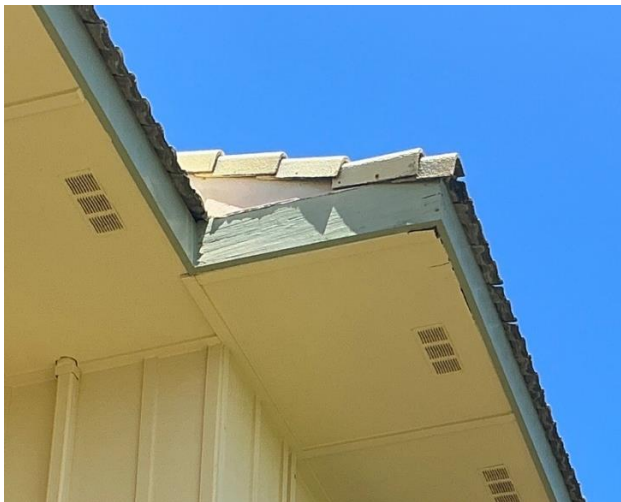
Figure 10. Typical corroded nails at the roof rake returns. Lihue elevation at Building D shown.
