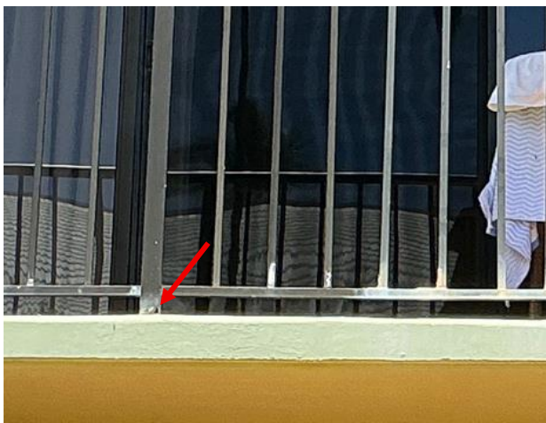
Figure 6. Hole at post unit E10 lanai
