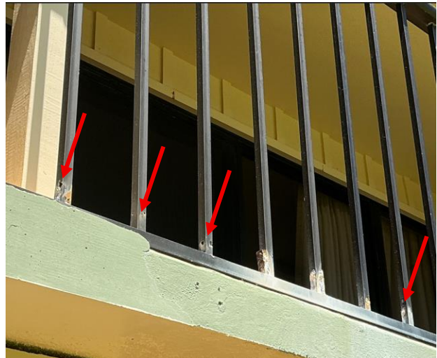
Figure 5. Typical Lanai Corrosion with full depth holes. Unit E10 shown.
