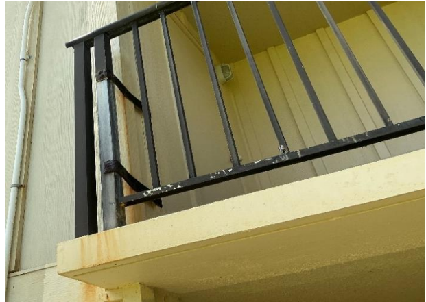
Figure 9. Corroded retrofit and full depth Holes due to Corrosion on Unit F3 Lanai
