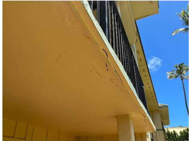
Figure 2. Overhead falling debris hazard unit E16
