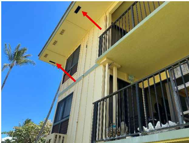
Figure 12. Missing vent covers at Building A. Condition is similar at other locations.
