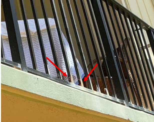
Figure 8. Corroded angle retrofits installed at railing pickets at Lihue elevation of Building D.
