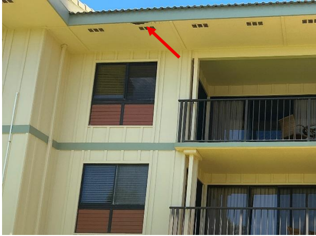
Figure 11. Decay of soffit panel at Lihue elevation of building D.
