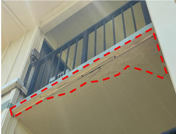
Figure 1. Overhead Falling Debris Hazard, Unit A17.
